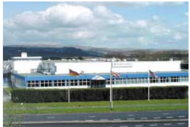
Barden's Super Precision Bearing plant located in Plymouth, Devon, U.K.
