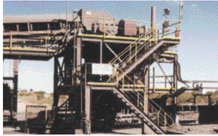
Conveyor plant drive unit
